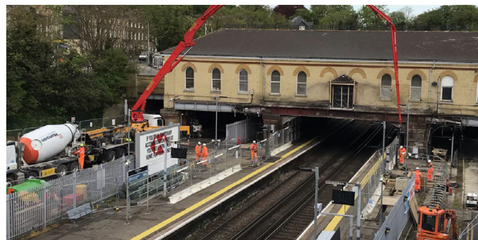
UK's largest single pour of an innovative new cement-free concrete at Chatham Station in Kent.
