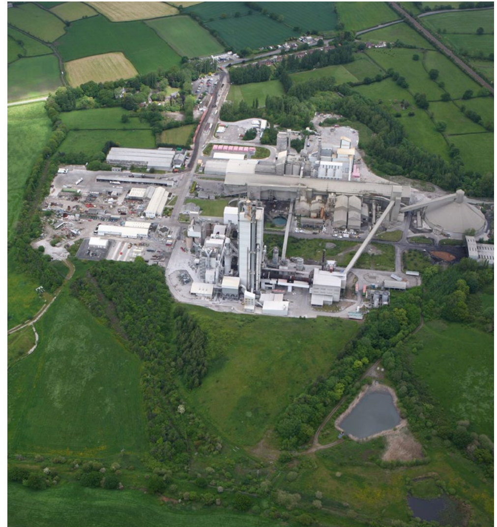
Padeswood cement plant in Mold, Flintshire
