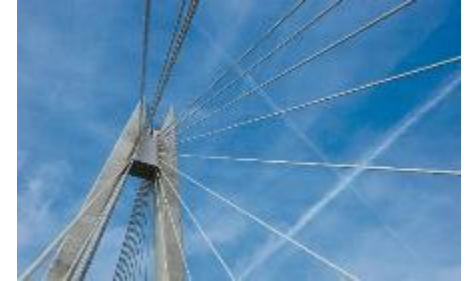
Bridges: Second Severn Crossing linking England and Wales
