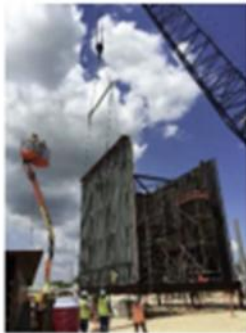
Box built up of Steel Panels
