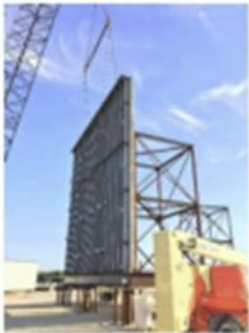
Preparation for Assembly of Steel Panels
