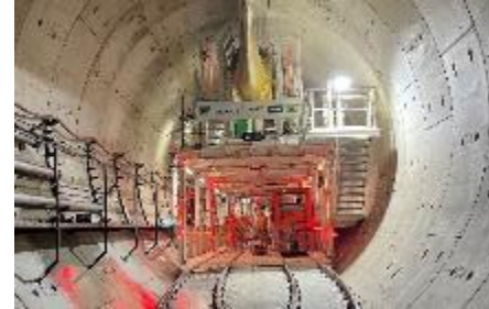
Tunnels: Thames Tideway super sewer, London
