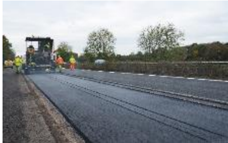
Roads: A414 resurfacing works, Hertfordshire
