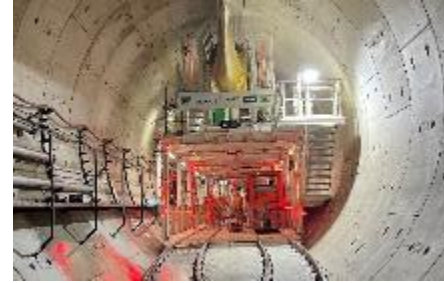
Tunnels: Thames Tideway super sewer, London
