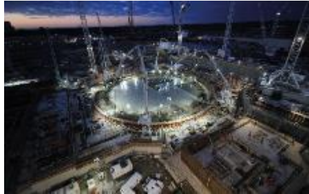
Power generation: Hinkley Point C, Somerset
