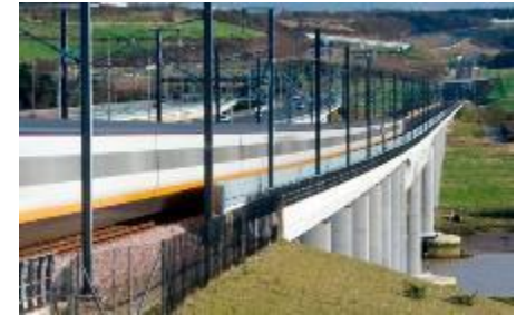
Rail: Channel Tunnel rail link
