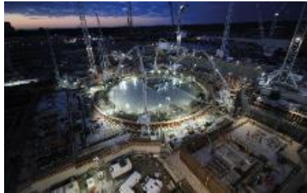
Power generation: Hinkley Point C, Somerset
