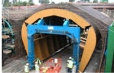
Dublin Port Tunnel Eire
