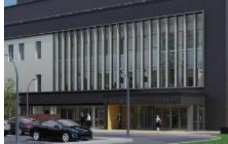
Hospitals: Christie Hospital, Manchester
