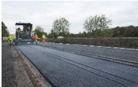
Roads: A414 resurfacing works, Hertfordshire
