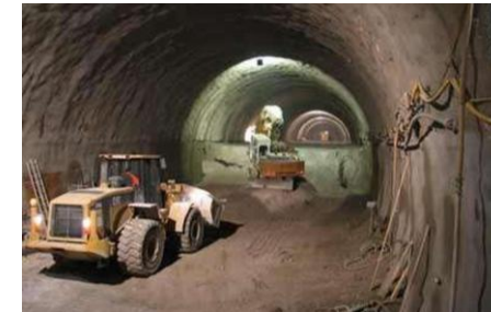
Brenner Rail Link Austria
