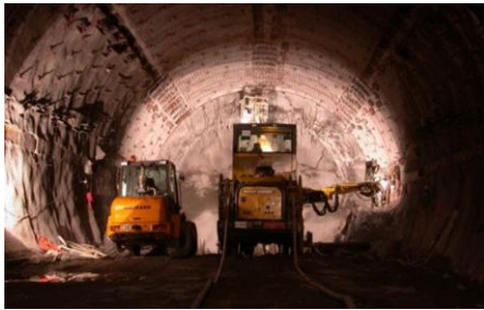
Gotthard Base Tunnel Switzerland
