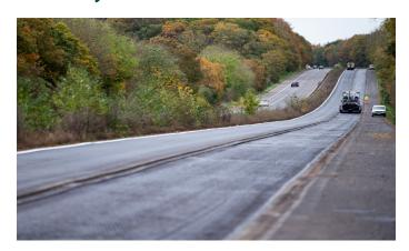
It was produced and laid at a lower temperature using Heidelberg Materials' ERA warm mix process, which reduces energy consumption and associated carbon emissions by up to 15 per cent. As a result, the production of the 940 tonnes of LT R used on the project generated a carbon saving of 2,246 kg of CO2 – the equivalent of driving more than 51,000 miles, or twice around the world.
