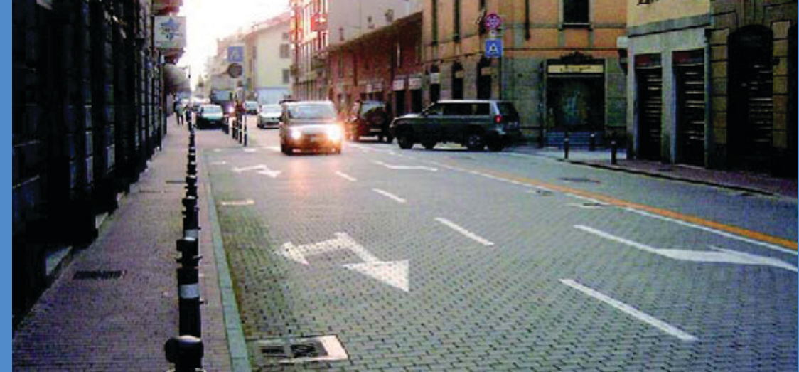
Borgo Palazzo Street, Bergamo, Italy with photocatalytic concrete block paving.
